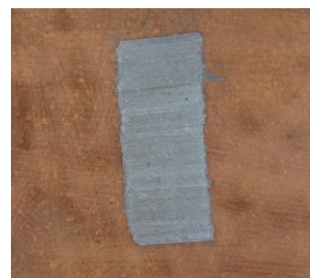
Heavy rust cleaning
